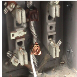
Step 2b Split-nut Ground Installation
