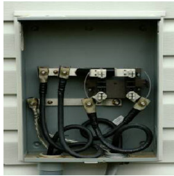
Step 2a Hi-Lug Ground Installation
