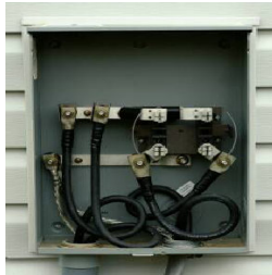
Step 2a Hi-Lug Ground Installation
